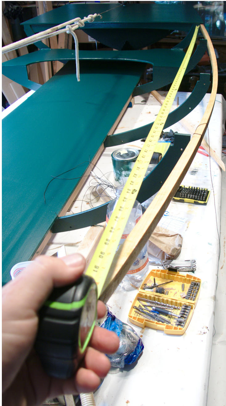
Figure 5.1. Check for the correct length before bolting the gunwales
